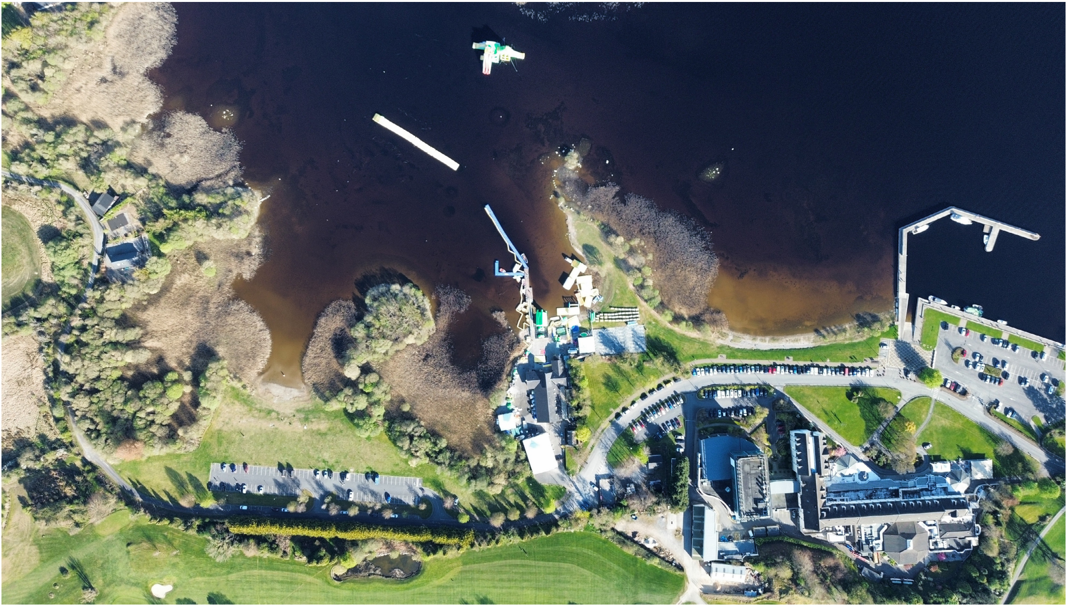
Site drone photo
